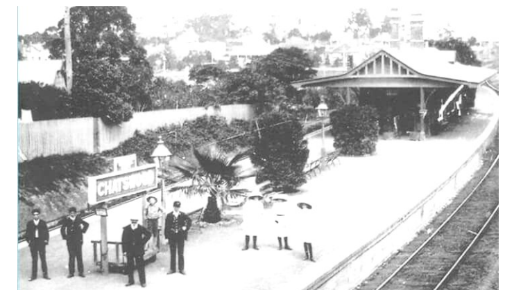
Chatswood Station 1900s
